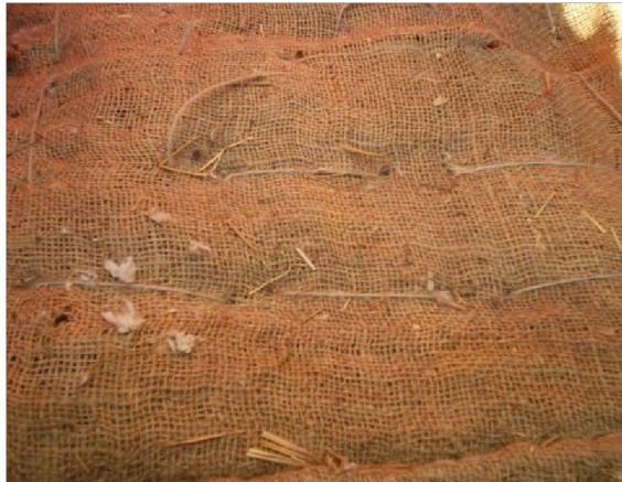
Picture 6.14: Sewing stuffing material put to spiral arch
