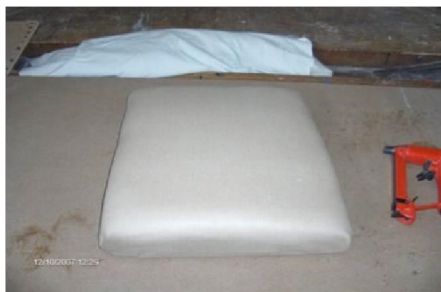
Picture 5.19:Placing fibe on the lining cloth
