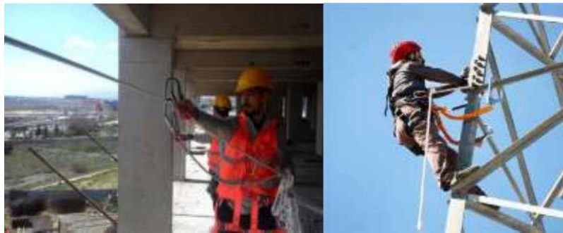
protective equipment against falls from height Photo 1.7
