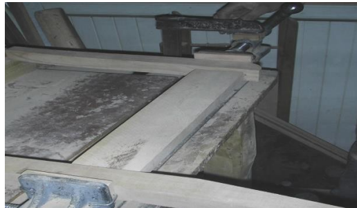
Picture 1. 3: Securing the rail restraint
